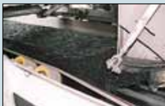
Soft loading – note the low impact angle of the coal stream landing on the belt.
